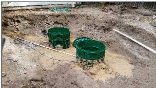
AK500F during installation
