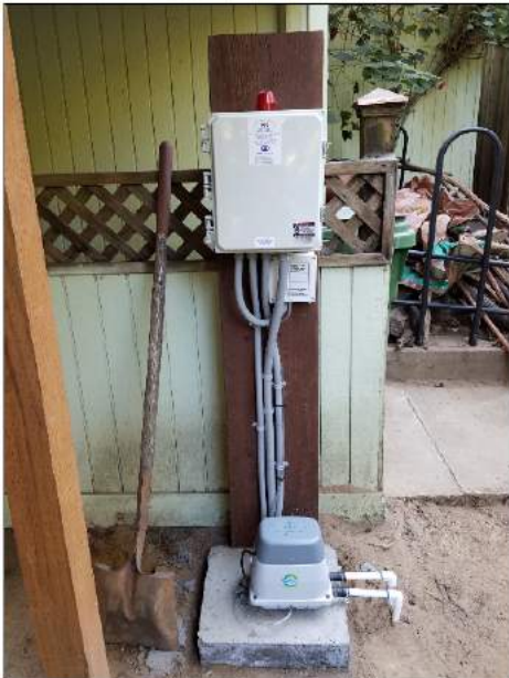
AquaKlear's control center (top to bottom): AKE Drip Controller, Rmsys monitoring system, AK Dual Outlet Compressor
