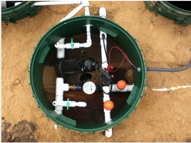
AquaKlear's headwork's manifold features a 120 micron disc filter, sampling port, flowmeter, solenoid valve & air-release valves (to prevent siphoning)
