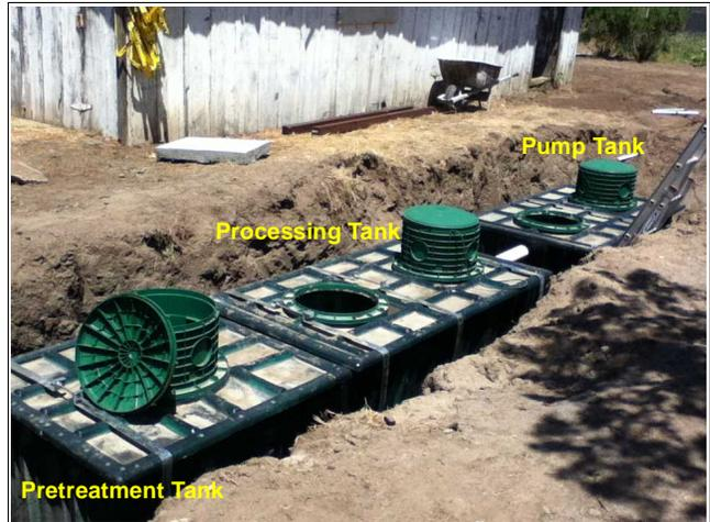
AK6S245F features a 424 gal pretreatment tank with 600 gpd processing unit; flows to separate 750 gal pump tank
